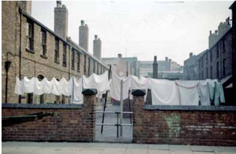
Photograph of 'improved' back-to-back housing (i.e. with the front of the court removed for better ventilation), known locally as 'Nettlefold Courts' after the chair of the Housing Committee, John Sutton Nettlefold, in Princip Street, off Loveday Street, adjoining the Gun Quarter. The photograph was taken in early 1960.
