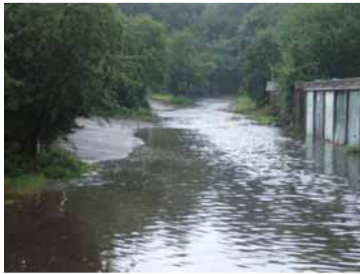
Site A Flooding and the proposed location for new houses.
